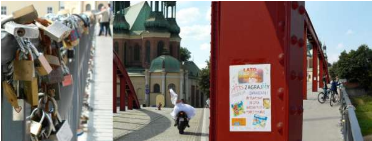
Fig. 3. The bridge linking Śródka with city centre (Photo: L. Podbrez, Poznań)
